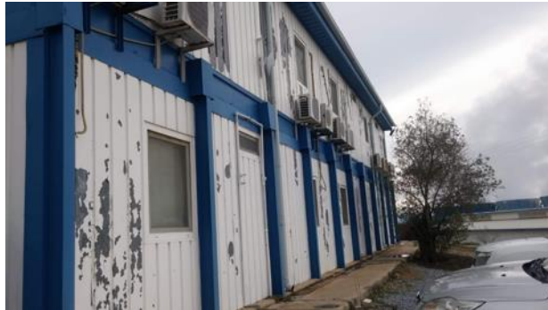
Photo 4-2. A Room in the Workers' Accommodation Building
